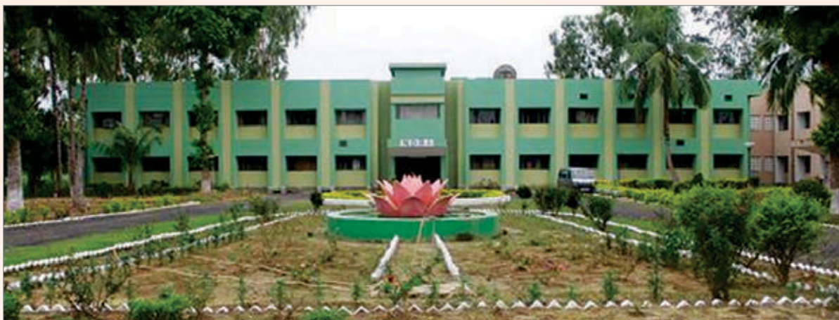
A view of ERS Building, Kalyani
